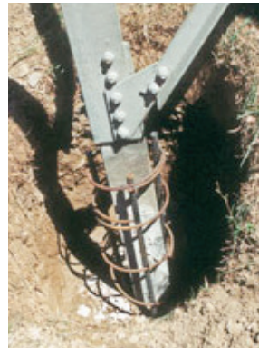
Repair in Progress
