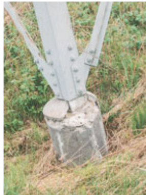
Damaged Foundation
