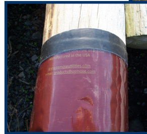
The liner is non-biodegradable and designed to resist the rigors of installation and backfilling.
